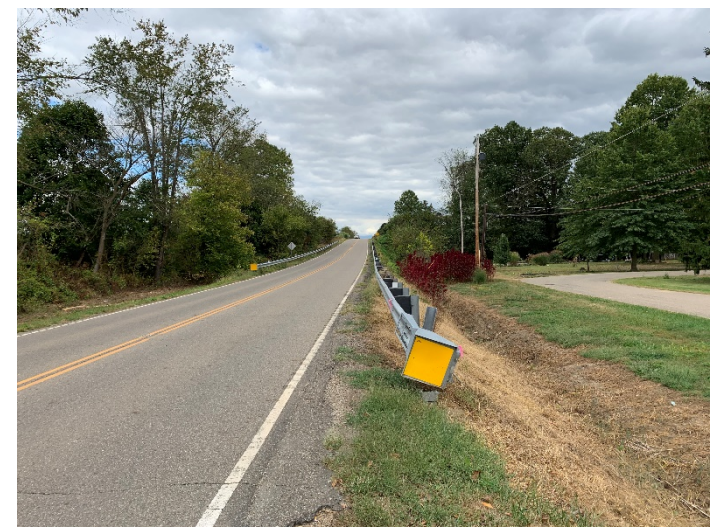
18. County Rd 16, looking E along water line alignment.
