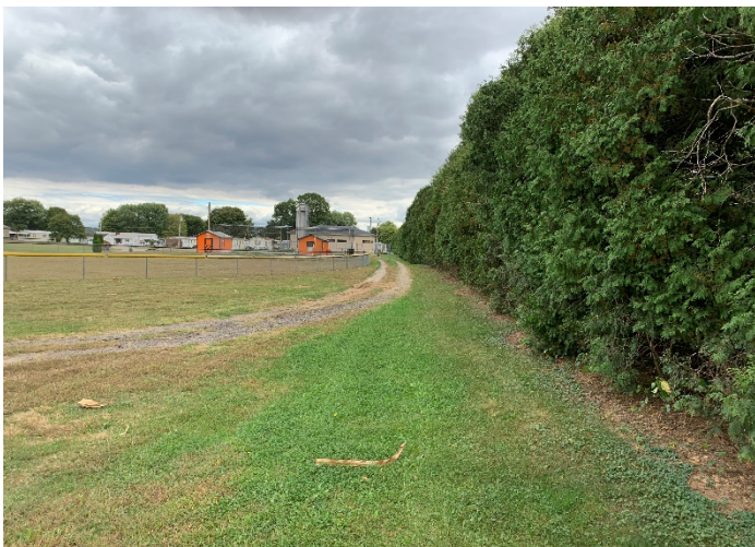
29. Final approach to Water Treatment Plant, looking E.
