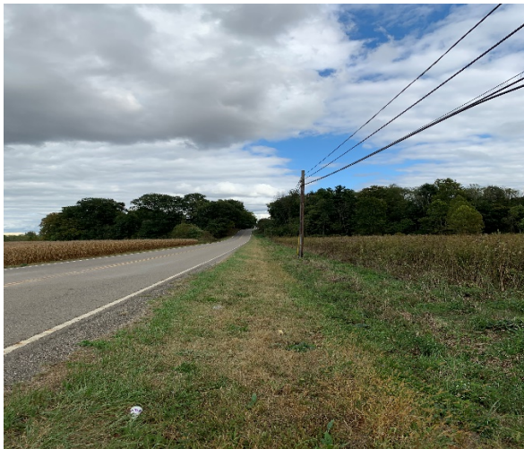
9. County Road 16 (looking East) along Pipeline Alignment.
