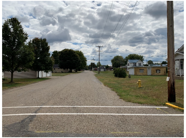
32. W. Lafayette Low Pressure Area, looking S along Gay St.
