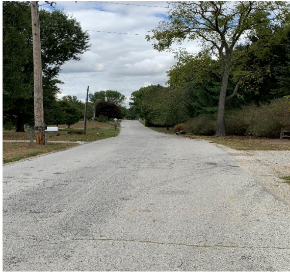
21. Area #3 looking W.
