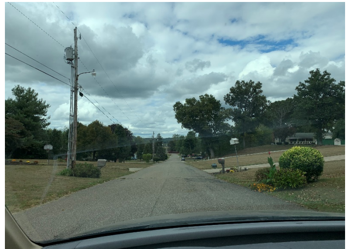
16. Area #2, looking South along water line alignment.
