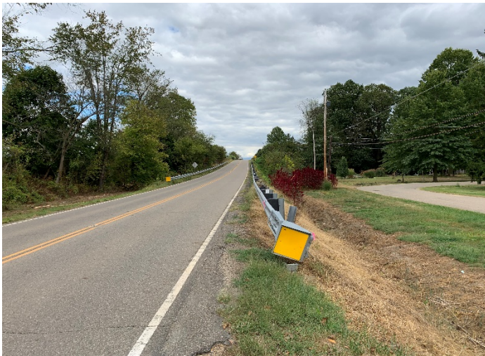
15. County Rd 16, looking E along water line alignment.
