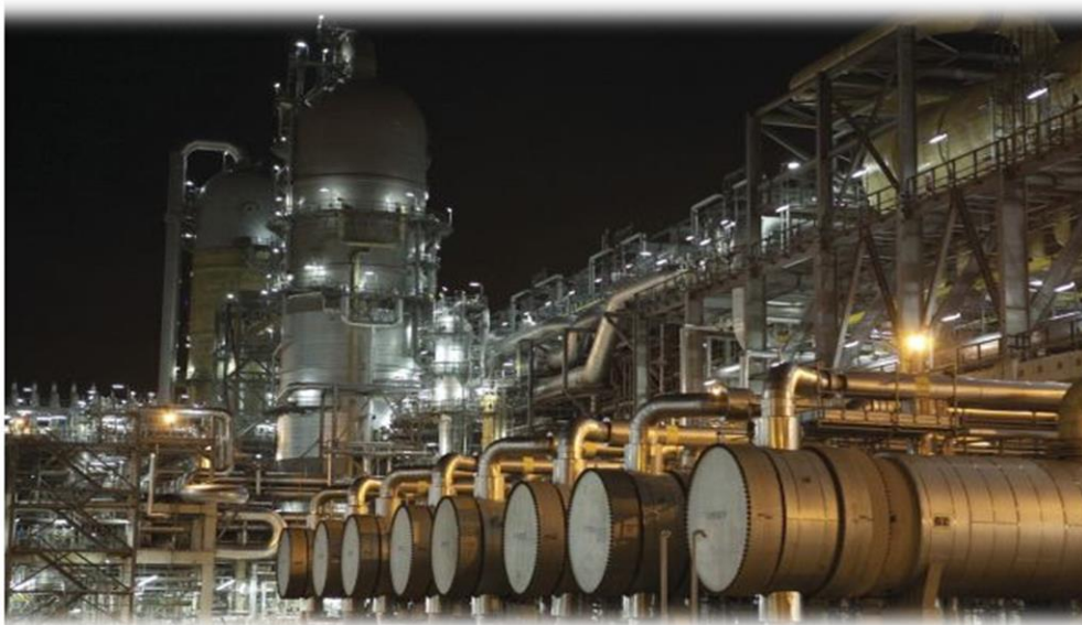
The proposed plant, similar to this one in Singapore, breaks ethane down into a substance that can be used to make chemicals and plastic. Ethane is a byproduct of natural gas.
